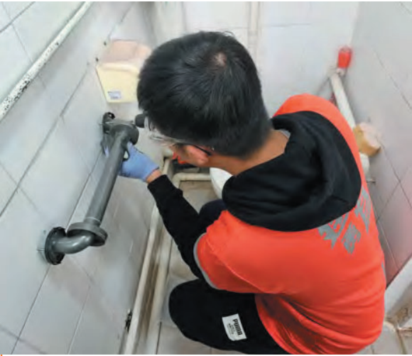
Construction Industry Volunteer Service Day - Construction Industry Volunteer Team installing handrails for elderlies
