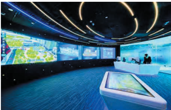
Smart Facilities Management Control Centre
